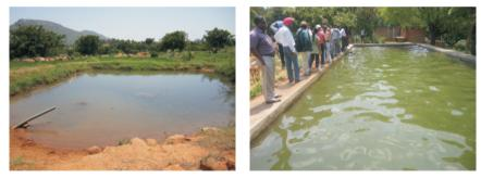
Unlined earthen storage structure (left) and cemented storage structure
